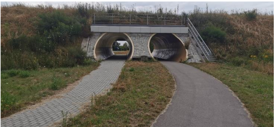
Figure 4. Pedestrian and bicycle tunnel at DW 815
