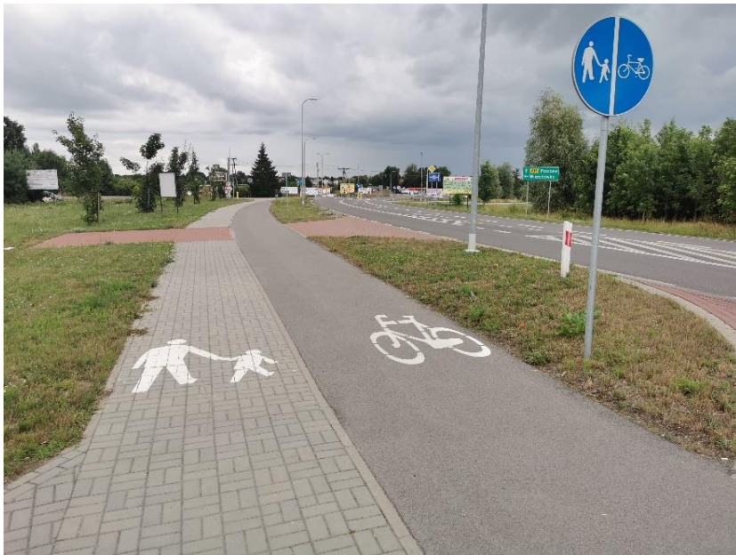
Figure 3. Pedestrian and bicycle route along DW 815 in Lubartów
