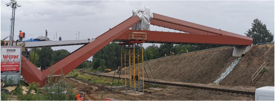
Figure 7. Construction of a footbridge in Lubartów
